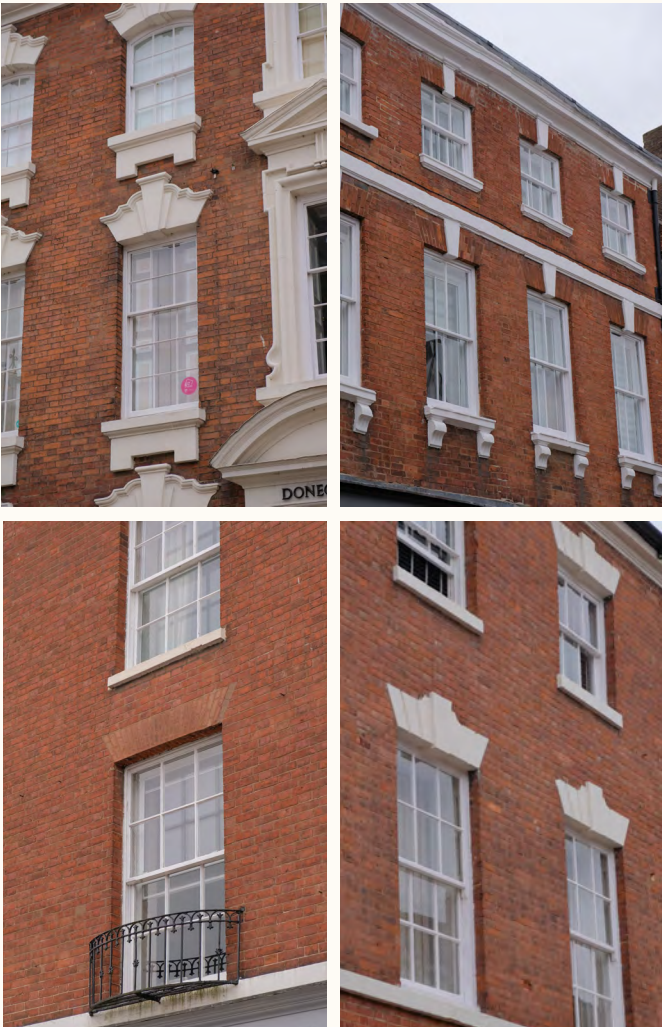
A selection of lintels from Lichfield: Baroque, flat gauge, and flat-gauge with masonry keystones.
