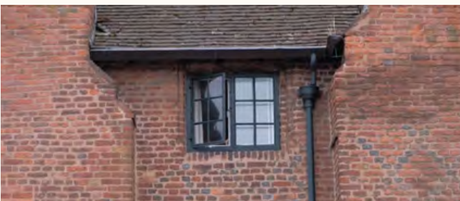
Left: A 2-over-2 sash window; Right: a bay window; Bottom: a casement window on St John's Hospice.
