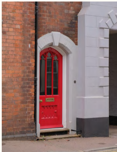
Left: Four-centred arch. Centre and Right: Victorian design saw Gothic motifs, such as masonry dressings and 'Venetian' arches.
