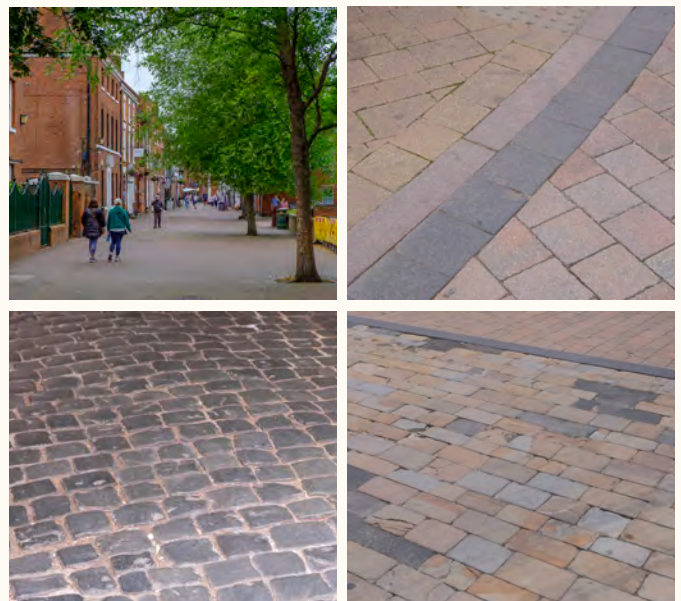
Clockwise from top left: shared surface on a traffic-free commercial street; a variety of clay pavers help delineate the carriageway; granite setts; clay pavers can be used on raised pavements too.
