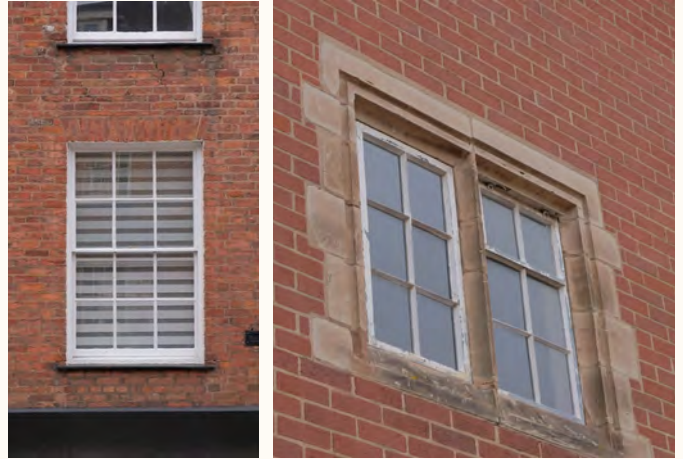
Left: A 6-over-6 sash window; Right: a casement window with masonry surround.
