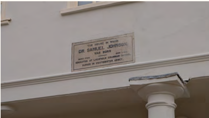
Render must be a smooth 'float' finish, and be of lime-base or stucco.
