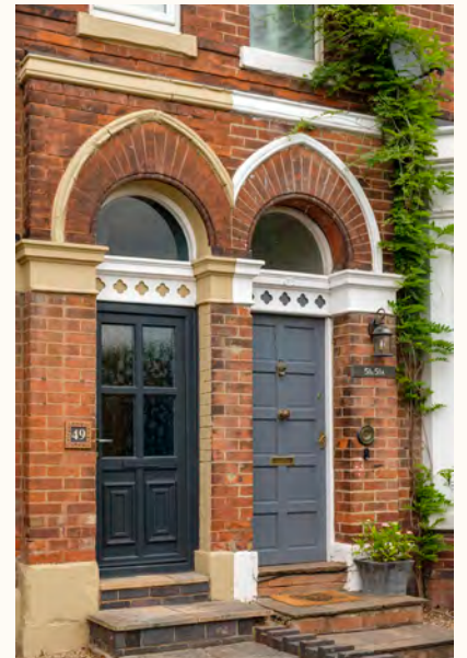
Left: Four-centred arch. Centre and Right: Victorian design saw Gothic motifs, such as masonry dressings and 'Venetian' arches.
